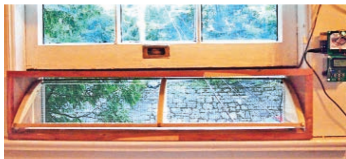
■ FIGURE 4: Inside view of a vent box and the controller.
